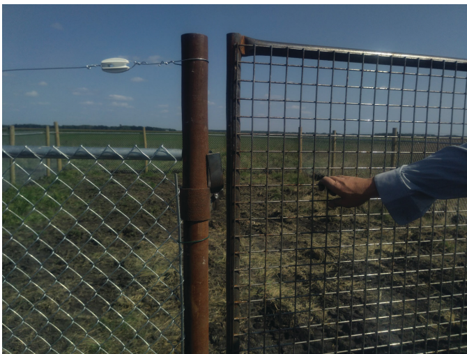
Tight fitting gate with chain link fence and high tensile top wire.
