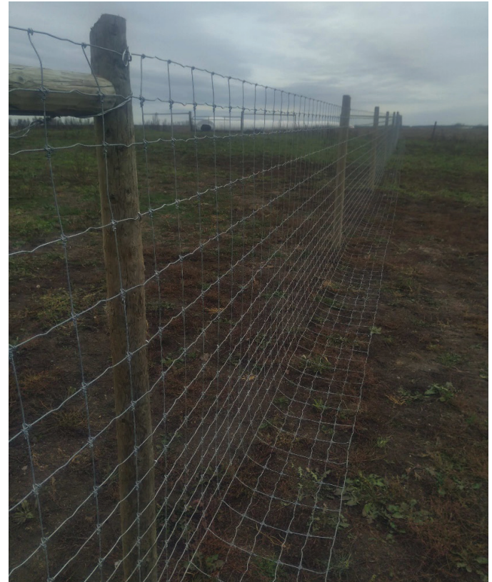
Example fence using Stay Tuff 868 apron wire hi-tensile fence. Note 22 inch apron on the ground.
