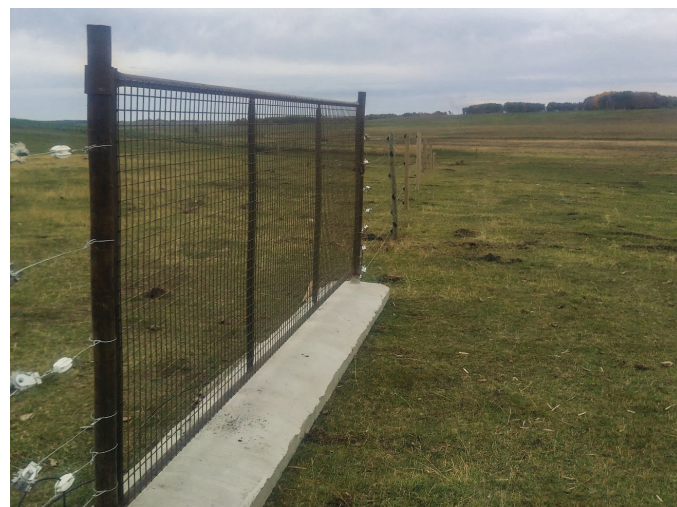
Pilot project predator resistant gate with 2 inch welded mesh, and tight fitting corners.
