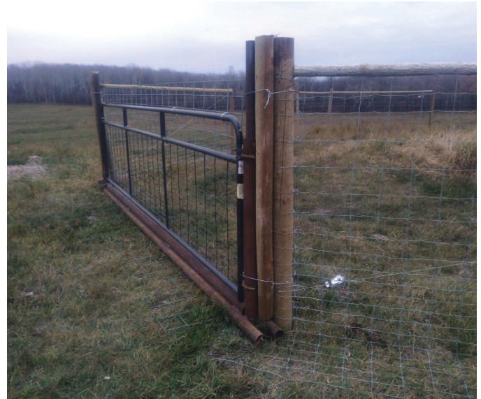
Predator resistant gate with drill stem threshold and hog panel as a dig-proof base.
